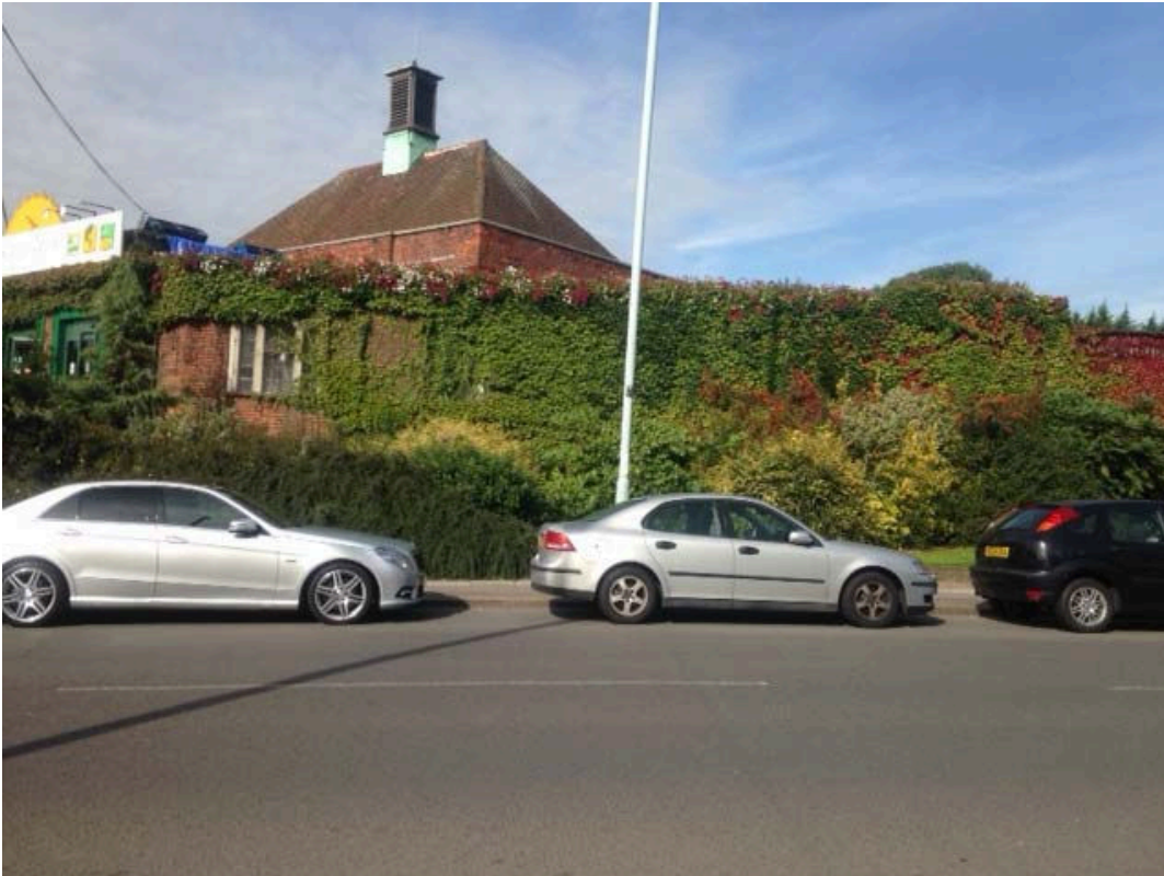
Central building viewed from Durnsford Road
