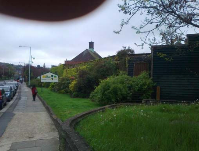
View of timber boarding façade from Durnsford Road
